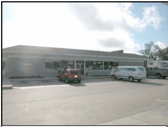
Figure 2: View of the convenience store looking eastward.
