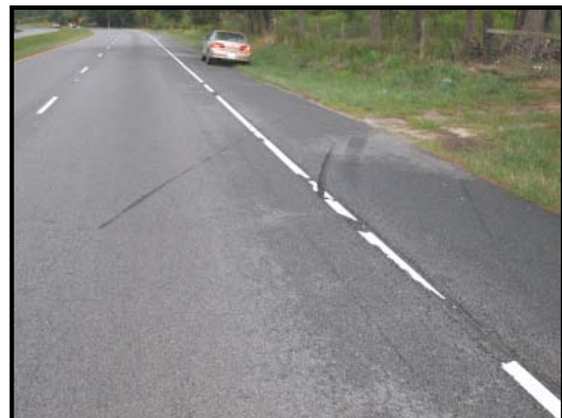
Figure 3: Physical road evidence of the vehicles' trajectories.
