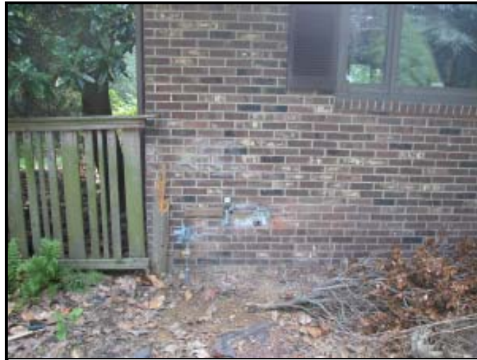
Figure 4: View of the point of impact
