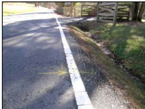
Figure 4. Roadside departure showing gouges
