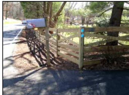
Figure 2. View of replaced fence, mailbox, and struck tree
