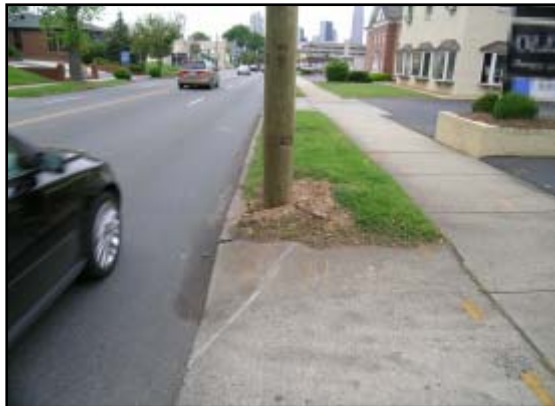
Figure 4. Second utility pole impact.
