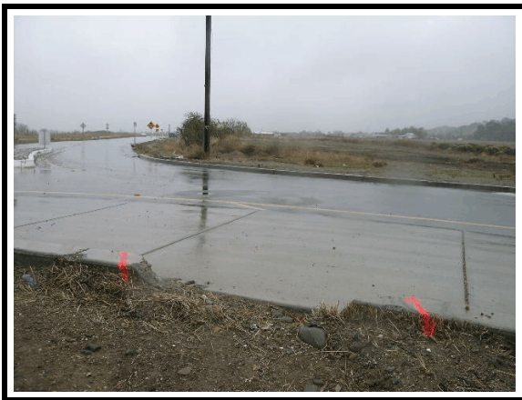
Figure 6. Damage from second curb impact (east)
