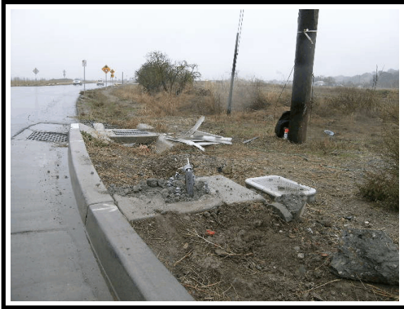
Figure 7. Pole sheared from its base
