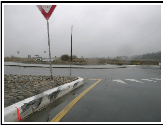
Figure 4. Initial roadway departure point and damaged yield sign (east)
