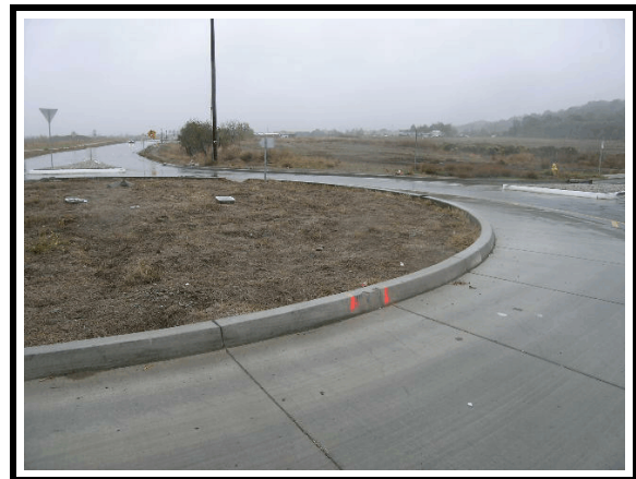
Figure 5. Damage to the traffic circle's inner curb (east)
