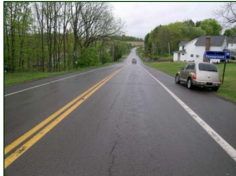
Figure 2. Northbound view of the crash site.
