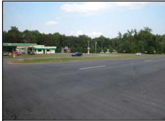
Figure 5. Final rest area for both vehicles.
