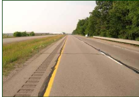
Figure 2. Northbound view of the crash site and the Venture's point of departure.
