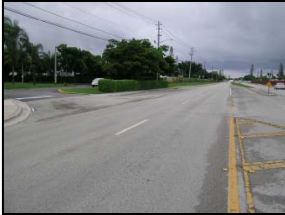
Figure 2: Northeasterly view of the crash site.
