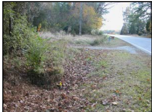
Figure 3: Trajectory view at the culvert.
