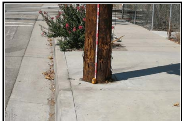
Figure 6. Impact with third pole
