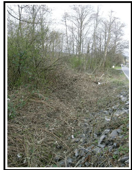
Figure 4. Ditch on west side of roadway; disturbed blackberry vines and damaged trees in background
