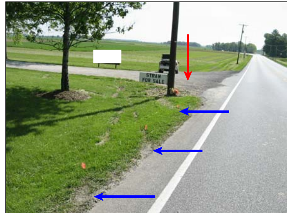
Figure 3: Overview of case vehicle's tire furrows (blue arrows) in grass and location of impacted utility pole, red arrow shows case vehicle's area of final rest
