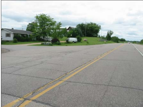
Figure 2: Approach of Kenworth southeastbound turning onto intersecting roadway
