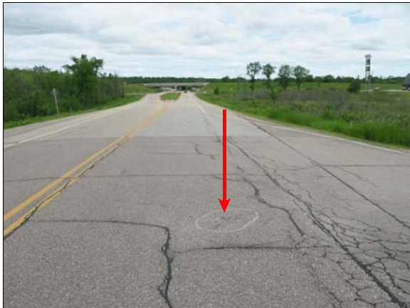
Figure 4: Approach of case vehicle northbound to impact, arrow shows impact gouges on pavement
