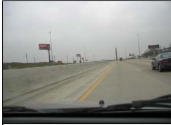
Figure 3. Approximate area of the median barrier impact, rollover, and final rest of the Ford.
