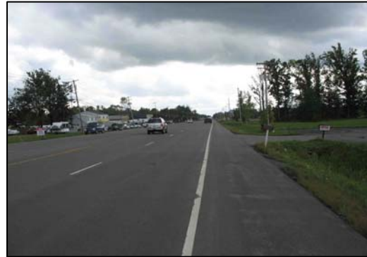
Figure 2 - Southbound approach of the Cavalier.
