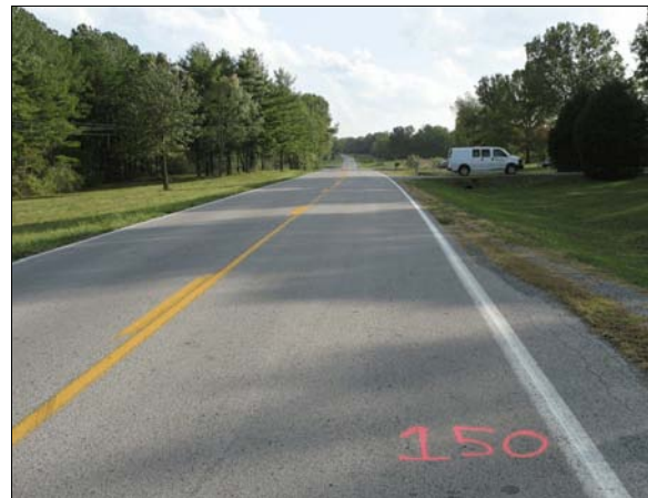
Figure 1: Pontiac's southbound travel path in slight left-hand curve; Pontiac drifted onto right shoulder before driver oversteered leftward, returning vehicle to roadway
