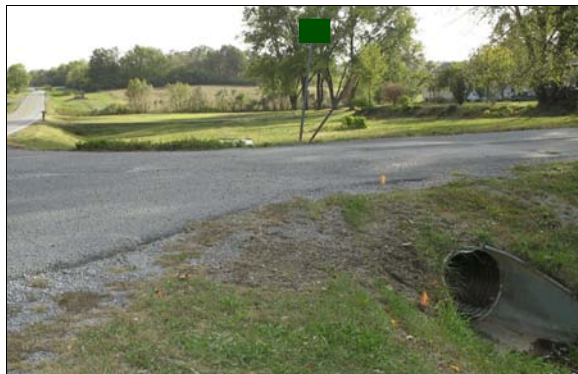
Figure 7: Pontiac's left front wheel impacts near culvert shearing wheel from vehicle and initiating vehicle's roll over
