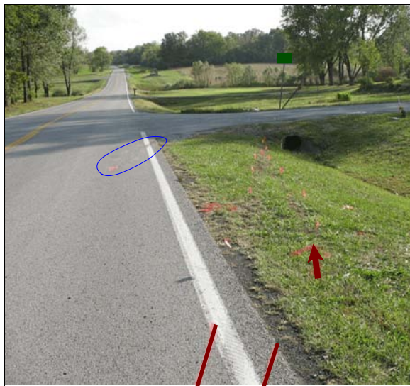
Figure 4: Pontiac’s travel path on south roadside toward culvert; scuff mark on south edge line from left front tire; arrow marks path of right front tire; highlighted area shows rear tire marks
