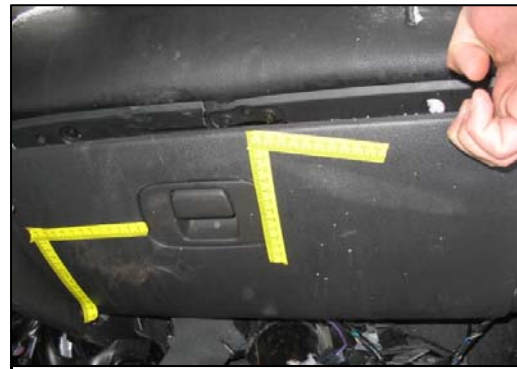
Figure 10 - Damage to glove compartment cover from front right passenger loading.
