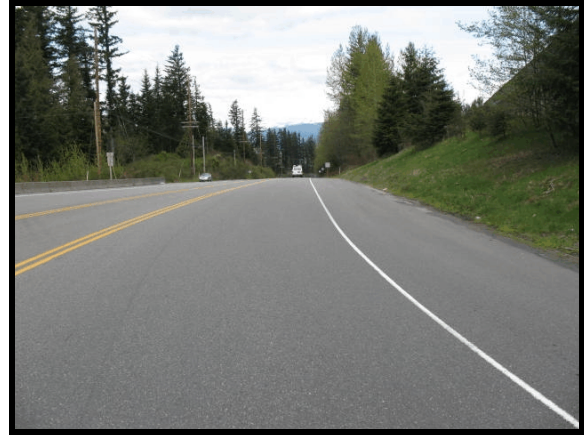
Figure 3. Eastbound approach to area of road departure and impact
