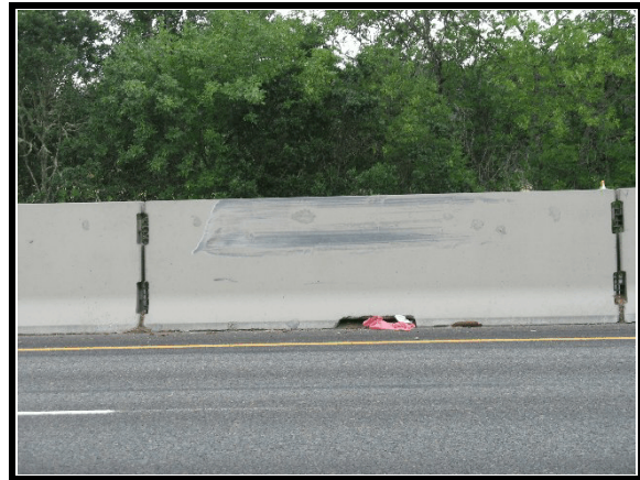
Figure 3. Evidence of trailer contact with center divider
