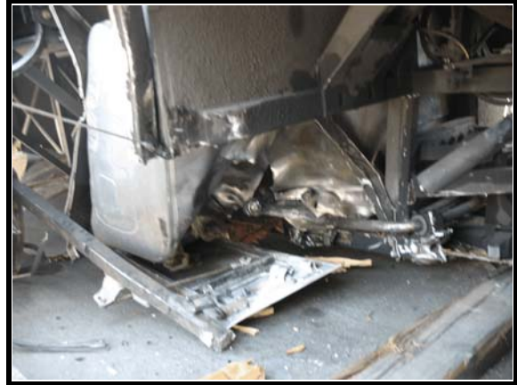
Figure 13. Fuel tank damage
