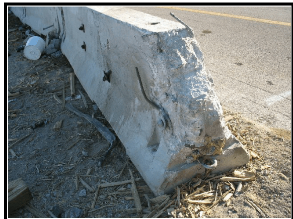
Figure 5. Struck concrete barrier
