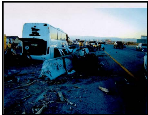
Figure 4. Area of impact, showing guardrail and concrete barrier (police photo)
