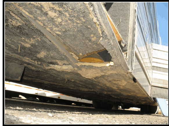
Figure 11. Damage to area below storage compartment
