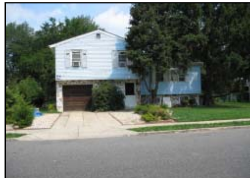
Figure 2. Overall view of the incident site.
