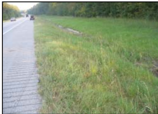
Figure 3. Overall view of the embankment where the Ford rolled over.
