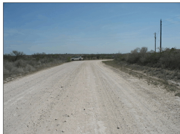
Figure 2: Approach of the Honda south to the area of roadway departure in the right curve
