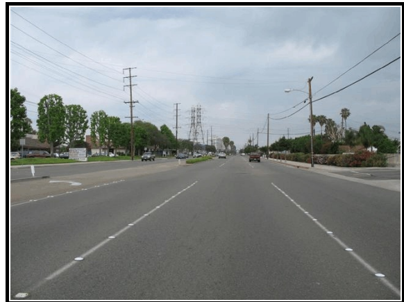
Figure 4. East leg of intersection
