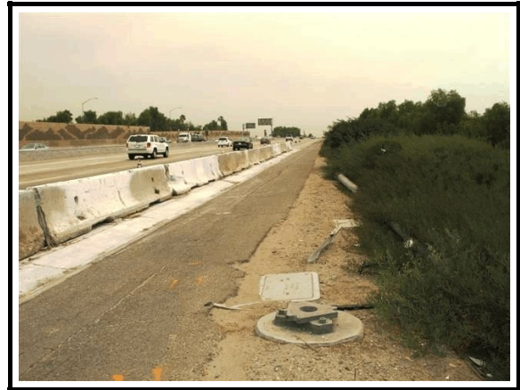
Figure 3. Point of impact with streetlight pole, base in foreground
