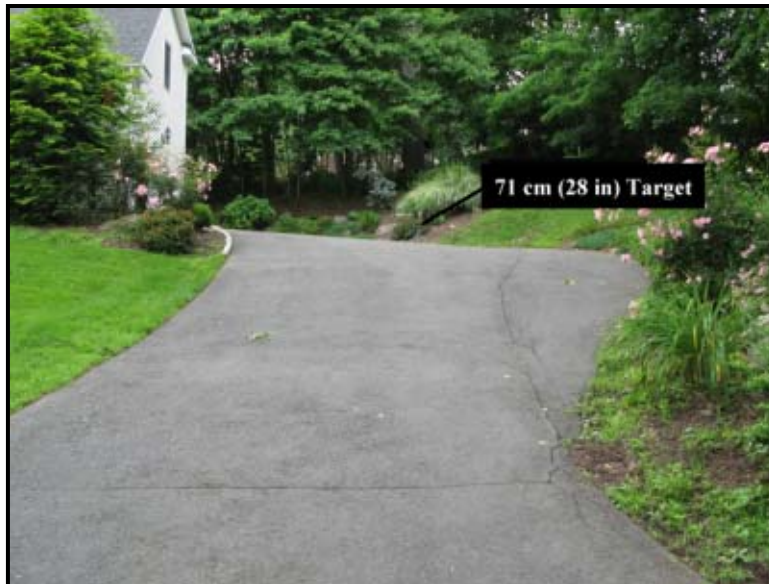
Figure 6: View from the base of the driveway with the 71 cm (28 in) target at the non-motorist location.
