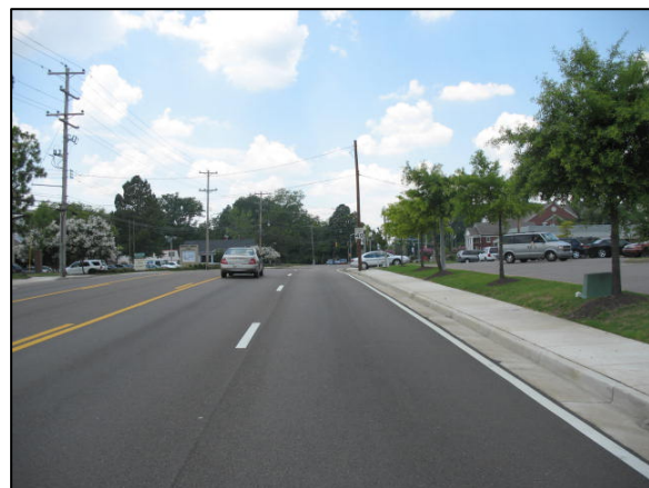
Figure 2: Westbound view of the GMC's pre-crash path of travel
