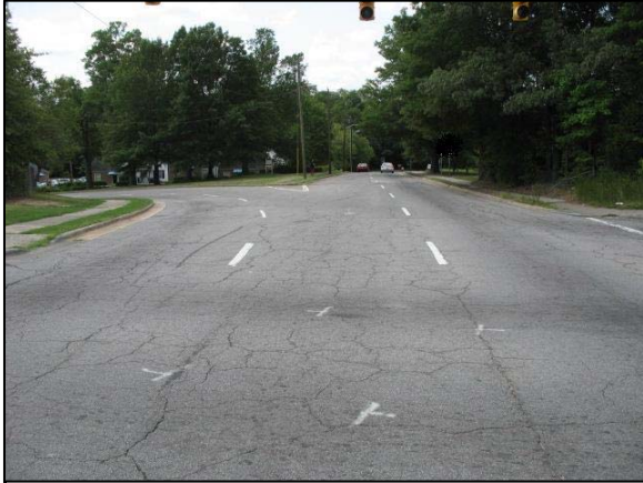
Figure 3: Southbound trajectory view of the area of initial impact.
