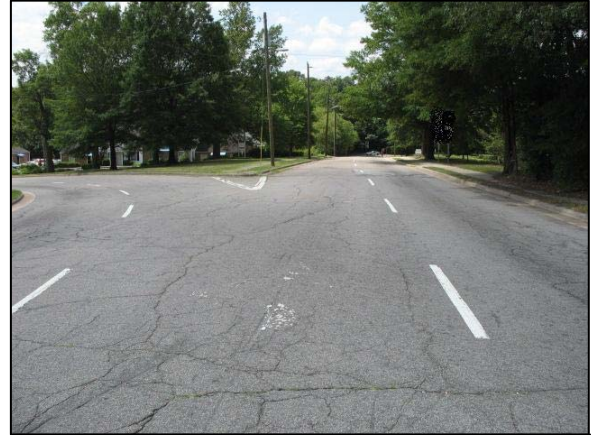
Figure 4: Southbound view at the location of the Toyota rollover.
