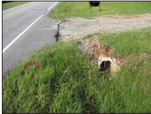
Figure 3: Westward view of the area of initial impact with the culvert.
