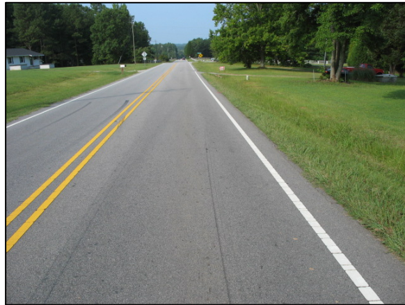
Figure 2: Westbound approach to the crash scene.
