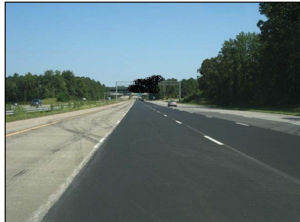
Figure 2: Northbound approach to the crash site.
