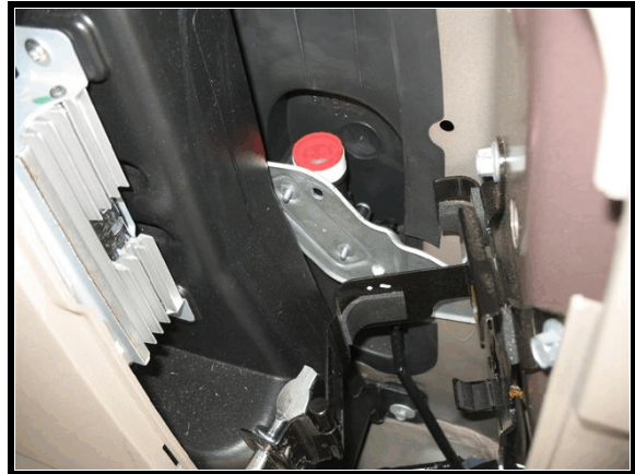
Figure 14. High-voltage shut-off switch
