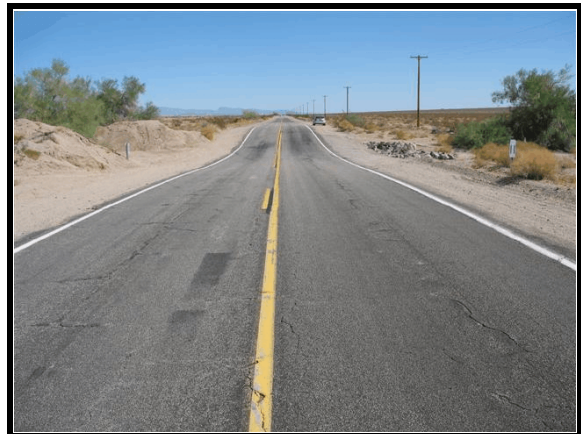
Figure 2. Eastbound approach showing sag in roadway
