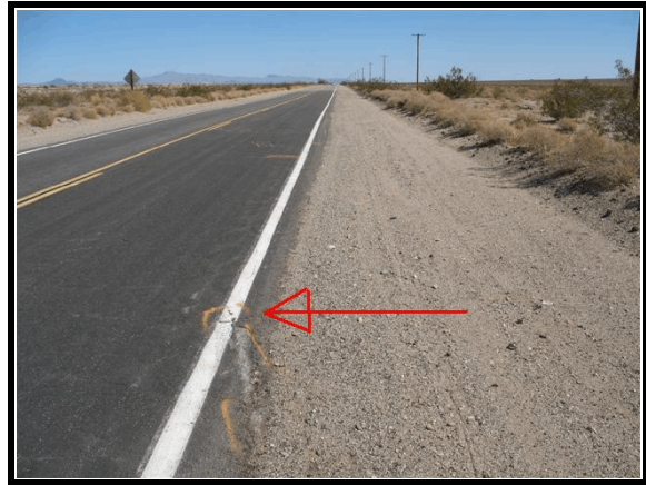
Figure 11. Trip point at junction of roadway and shoulder
