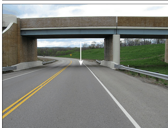
Figure 3: Approach of the Ford; arrow shows area of the impact
