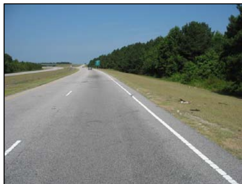
Figure 2: Overall westbound view of the crash site.
