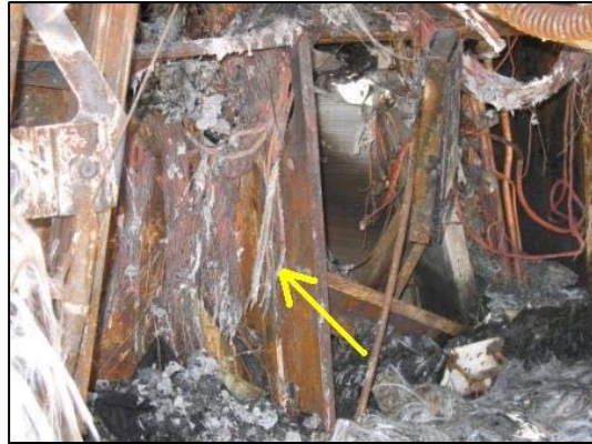
Figure 13. Right side panel box and the cable damage (arrow).
