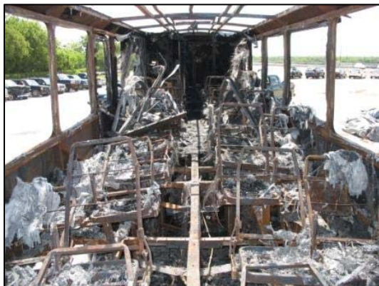
Figure 16. Rearward view of the interior fire damage to the motorcoach.
