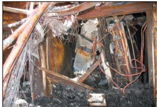
Figure 14. AC evaporators and related fire damage located aft of the luggage compartments.
