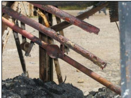
Figure 15. Example of the fire damage to the copper refrigerant supply and return lines.
