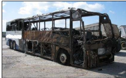
Figure 9. Right side view of the fire damage to the motorcoach.
