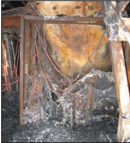
Figure 12. Left side panel box, wiring, and heat evidence.
