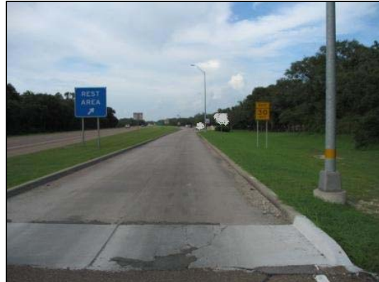
Figure 2. Northeasterly view of the off-ramp approach to the incident site.
