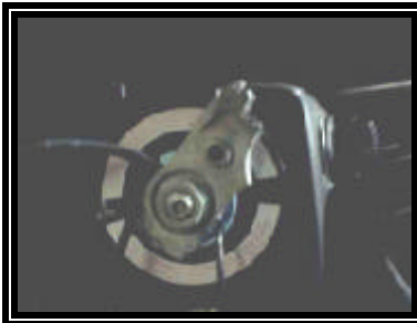
Figure 11. Close up view of fractured mounting bracket
