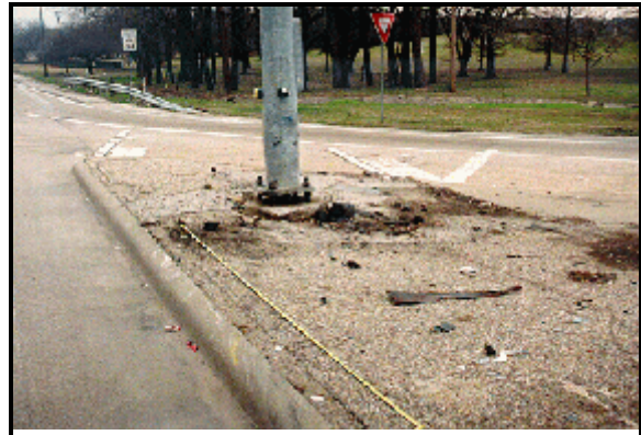
Figure 9: East-southeast view of traffic signal pole impacted by case vehicle's front located on traffic island off southeast corner of intersection (case photo #04)
