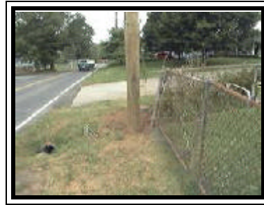
Figure 2. Utility pole impact location (pole replaced).
