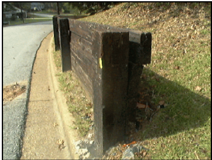
Figure 2. Wooden retaining wall (closeup)
