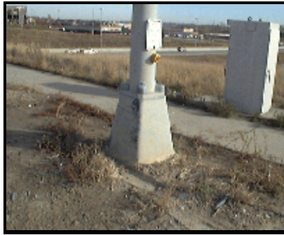
Figure 5. Impacted Traffic Signal Pole (Vehicle 2, Second Impact)
