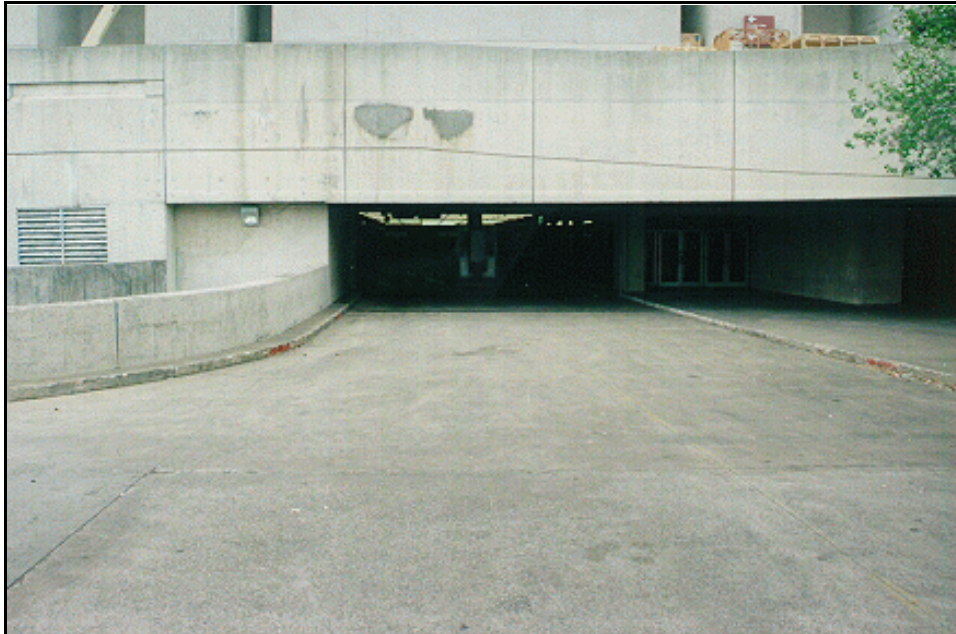
Figure 1: Case vehicle's eastbound approach toward impact with an overhead door that is raised in this view (case photo #1)
