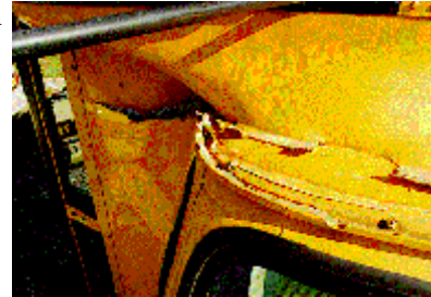
Figure 7. Fracture/separation of the fiberglass filler panels.
