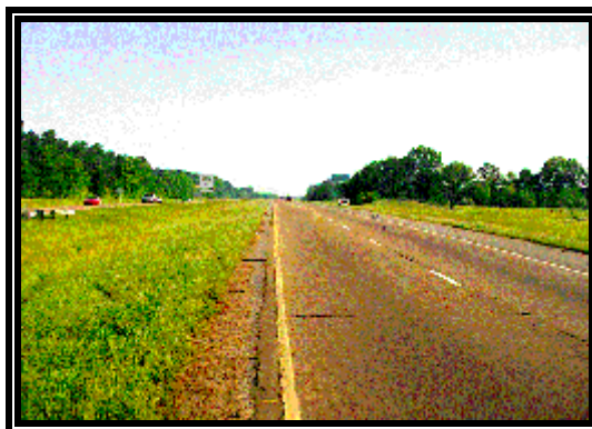
Figure 1: Northbound trajectory view of the interstate.
