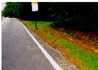
Figure 4. Point where the Toyota exited the roadway.
