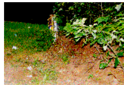
Figure 6. Close-up view of the fire hydrant and tree root.
