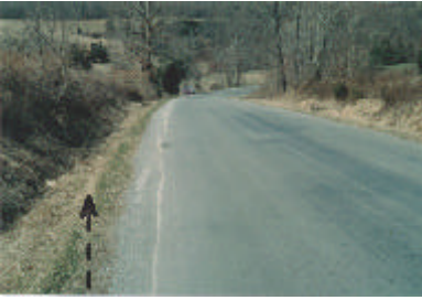
Figure 1 View of the vehicle's trajectory at the point of the first departure
