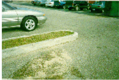
Figure 3- View of the curb showing impact evidence with the lower frontal area of the Plymouth
