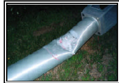
Figure 7. Fractured luminaire showing deformation and paint transfers
