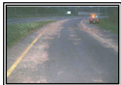
Figure 4. Point of impact looking northbound
